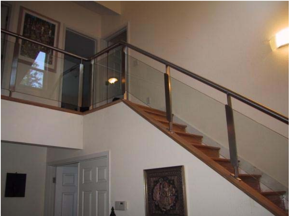
Custom built stainless steel railings with tempered glass.
